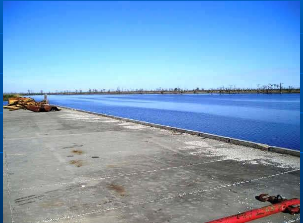
Empty barge dock at Port Manchac
