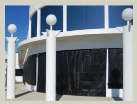
Figure 4-18. Polyethylene basket weave fabric windscreen deployed directly over ground floor windows of coastal home. Source: Roll-a-way/OMI.
