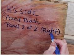
**Figures 4-21 and 4-22.** Not only is it necessary to install plywood opening covers correctly, it is also important to label them correctly and store them away from heat and humidity.
