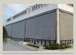
Figure 4-19. Polyethylene basket weave fabric windscreen deployed at edge of patio, enclosing the entire area. Source: Roll-a-way/OMI.
