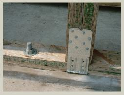
**Figure 4-27.** In some retrofit examples, it is possible to tie a portion of the house to the foundation. Here, a metal strap connects the vertical post to the foundation, which finishes the continuous load path connection from roof to the foundation. Source: Louisiana Sea Grant.
