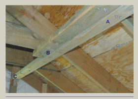
**Figure 4-7.** In this application of lateral bracing, the 2 x 4s are 18 inches from the ridge and connect to horizontal members that attach to the opposing trusses. Not all roofs will have the horizontal members. The 2 x 4s are connected with two No. 14 3-inch screws (A) and overlap over two trusses (A and B). The end is connected to the gable end with an angle or L bracket (C).
