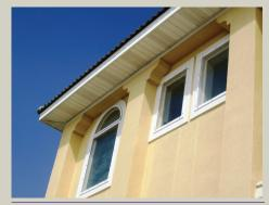
**Figure 4-17.** Flat impact polycarbonate panels installed directly over windows of a coastal home. This window covering provides excellent storm protection with minimal aesthetic impact. Source: Roll-a-way/QMI.
