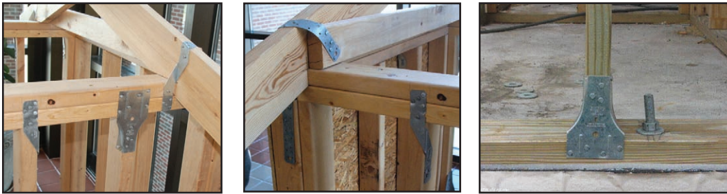
Figures 6-15, 6-16 and 6-17. In the LaHouse model home, hurricane straps are used to complete the continuous load path connection. The stud to single plate connector helps secure the house frame to its foundations and helps the home better withstand uplift. For new construction, the additional cost of implementing stronger connections may be minimal (Figures 6-15 and 6-16, photos by D. Hwang, 2007; Figure 6-17, photo courtesy of LSU AgCenter).
