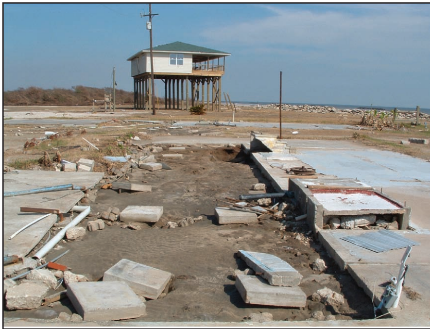
Figure 1-19. Constance Beach, Cameron Parish, Louisiana, after Hurricane Rita. While the house in the foreground was washed away by Rita's storm surge, the structure behind escaped destruction because it was properly elevated (Photo courtesy of D. Dartez, 2005).
