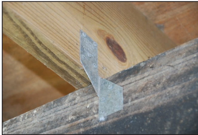
Figure 6-6. Existing home retrofitted with hurricane clips (Courtesy of LSU AgCenter).
