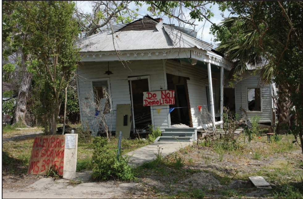
Figure 6-3. This home was forced off of its foundation by lateral loading (Photo by B. Kennedy, 2006).
