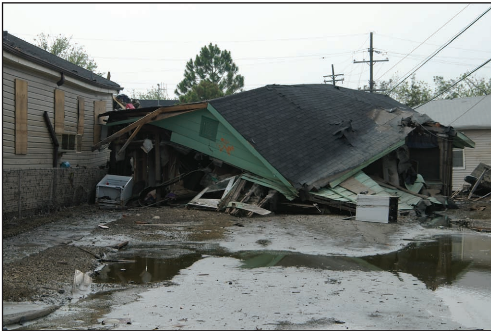
Figure 6-2. Air pressure and uplift worked to detach this roof from the rest of the structure. These types of forces can be mitigated against through the use of stronger connections, such as hurricane clips (Photo by B. Kennedy, 2006).
