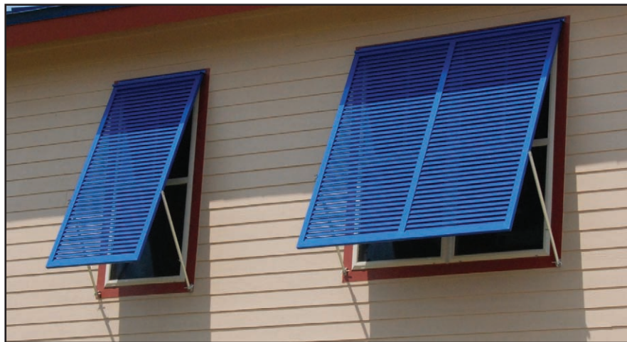
Figure 6-13. Permanently installed Bahama shutters provide light and shade when opened and protection from wind-borne debris when closed (Photo by D. Hwang, 2007).
