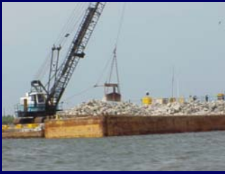
Building rock breakwaters to reduce wave erosion - Grand Isle, La.
