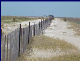
Sand fencing restores dunes on a barrier island - Terrebonne Parish.
