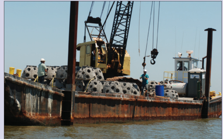
Reef balls being placed in Lake Ponchartrain to form habitat for fish.
