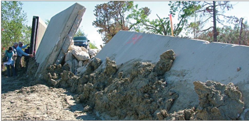
Displaced earth and concrete show that the forces of Hurricane Katrina were more than the London Avenue Canal floodwall in New Orleans could withstand.
