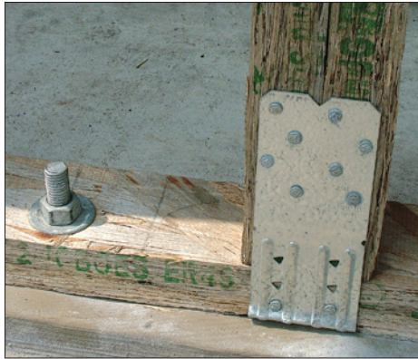
The addition of metal braces and brackets at strategic locations on the LaHouse frame gives the structure extra strength to withstand high winds, as Claudette Reichel (right) points out.
