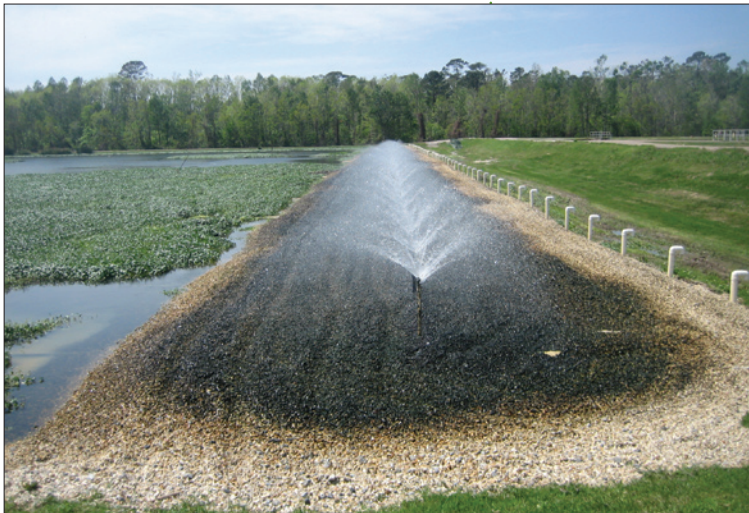
A three-celled rock reed filter is used in Mandeville's wastewater treatment process. Photo by Robert Lane.
