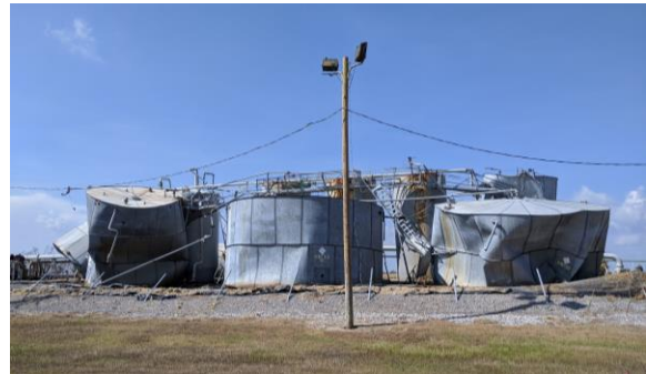
Figure 2. Damaged ASTs near Cameron, LA, after hurricane Laura (picture taken by the PI).
