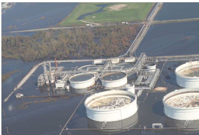
Figure 1. Flooded storage tanks at a chemical company in Jefferson Parish after Hurricane Ida (09/04/2021).
