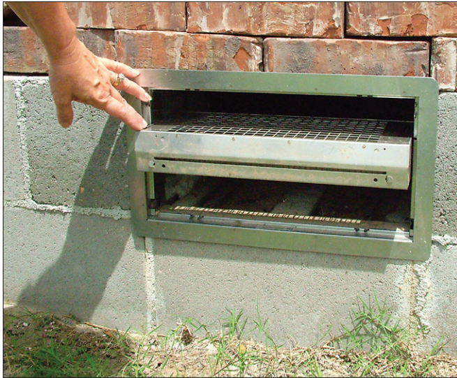
Flood vents allow rising water to pass in and out freely, reducing pressure that could cause a home's foundation to fail.
