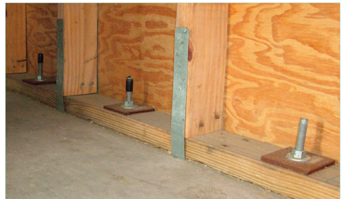
A series of straps and bolts anchor the house frame to its foundation, making the structure more wind resistant.
