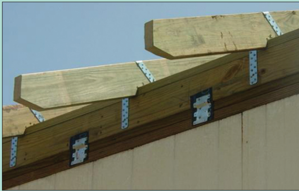
Hurricane straps more firmly affix the house's roof to load-bearing walls, resulting in the roof being less likely to blow off in high winds.
