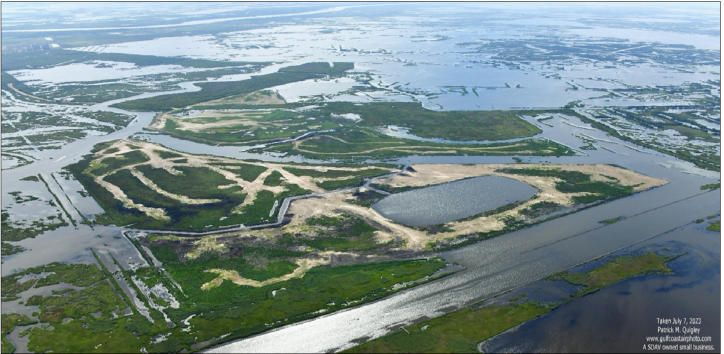
The Upper Barataria Marsh Creation project created 1,170 acres of emergent wetland habitat, 89 acres of water features — including a tidal pond and 18,815 linear feet of flow pathways that emulate natural tidal creeks, and strategic dike gaps that ensure water and wildlife can easily move between the new marsh and the larger basin. Credit: Patrick M. Quigley.
